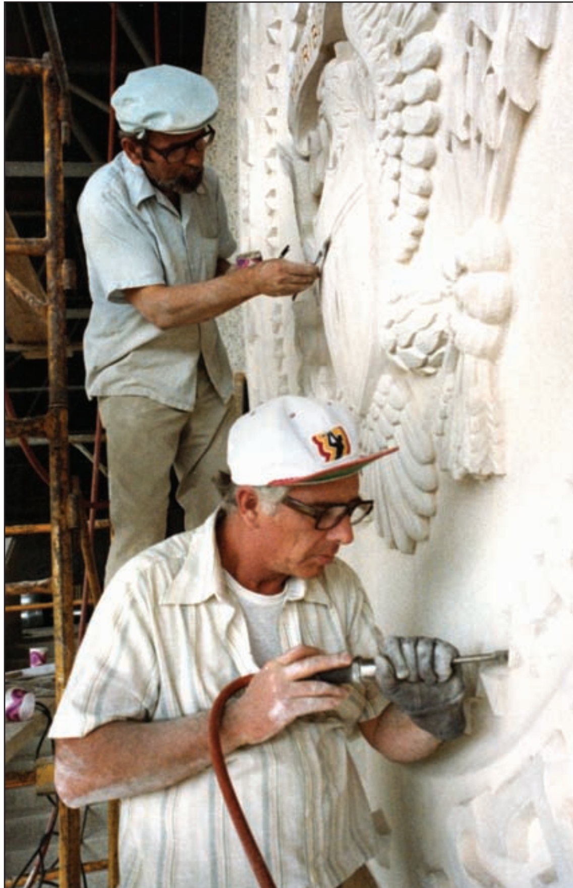
RIGHT: Harold Vogel (foreground) uses a pneumatic hammer to carve Indiana Buff Limestone Presidential Seal at Gerald R. Ford Museum in Grand Rapids, Mich.
