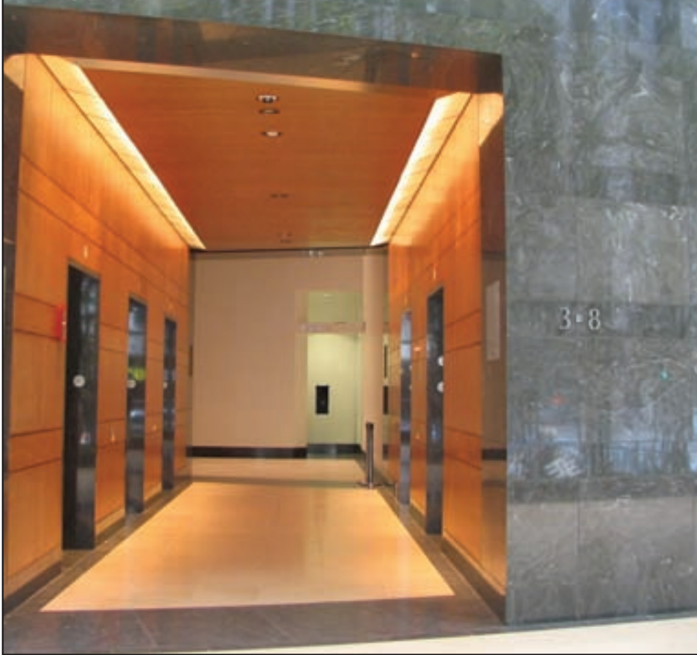
LEFT: At the Hyatt Center in Chicago, Virginia Mist granite was used for all of the interior and exterior wall cladding, paving, vanities and planters.
