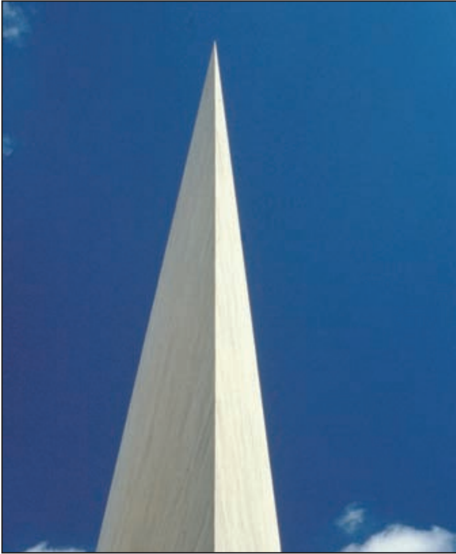
ABOVE: Possibly the sharpest corner of any building in the world, the East Building's signature "knife edge" cleaves the air at an angle of 19.5 degrees to a height of 116 feet.
